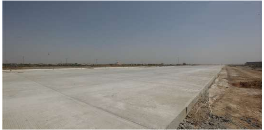
PQC (RIGID PAVEMENT) COMPLETED AT KM. 3
