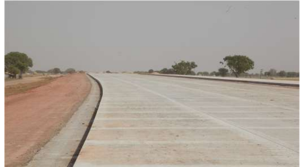
PQC (RIGID PAVEMENT) COMPLETED AT KM. 136
